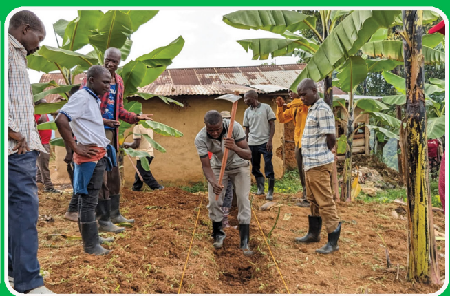
Elgon Communities learning how to make trenches
